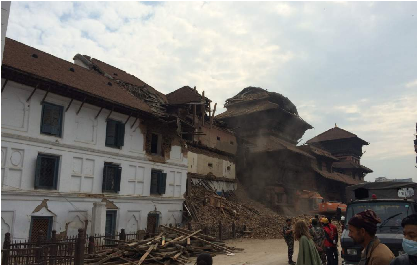
Fig. 6.1. Damage to Durbar Square from the Kathmandu Earthquake
