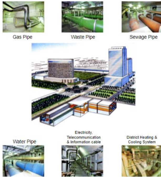
Figure 2. Utilidor in Tokyo Waterfront City in Japan
