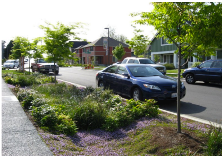
Figure 8. Urban bioswales can absorb significant amounts of excess stormwater and associated pollutant runoff. Source: Courtesy of the U.S. EPA.
