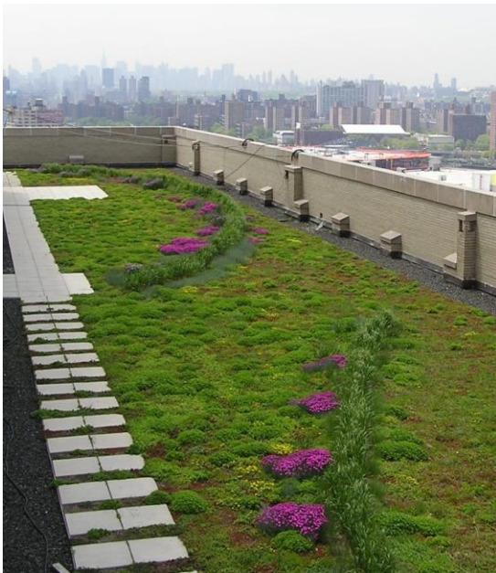
New York City green roof. Credit: Gowanus Canal Conservancy
