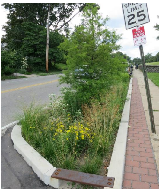
Stormwater Bumpout. Credit: Philadelphia Water Department
