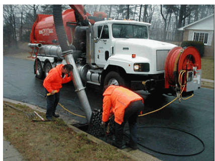
Figure 7. Storm drain facility cleaning (Source: Anne Arundel County, Maryland).
