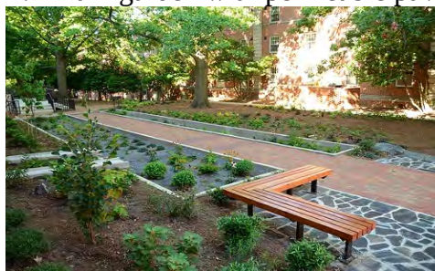
Figure 1: A rain garden with permeable pavement 43
