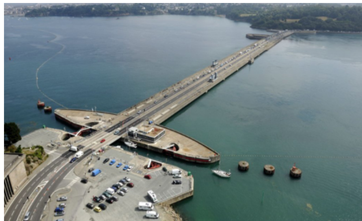
Figure 14: In the photo above is the La Rance tidal barrage in France that generates electricity twice a day from incoming and retreating tides. Image source: Energy BC 74
