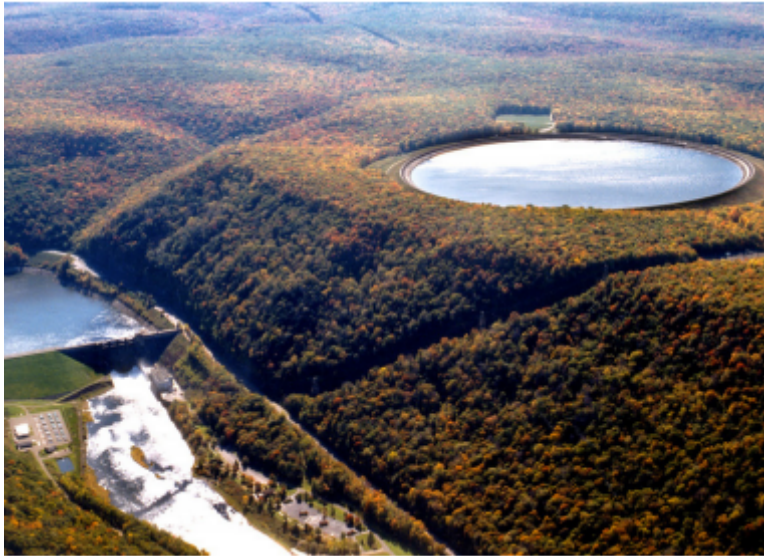
Figure 11: Pumped storage facility at Seneca, Pennsylvania. Image Source: RTO Insider 41
