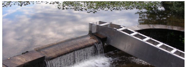
Figure 12: A fish ladder near the south shore of Long Island, New York that assists with the Alewife migration over the infrastructure of the dam. Source: NOAA 66
