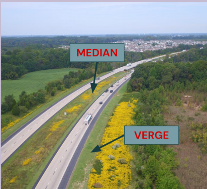
Figure 9: Image depicting a roadside median and verge. Image from (Delaware Department of Transportation, 2018).
