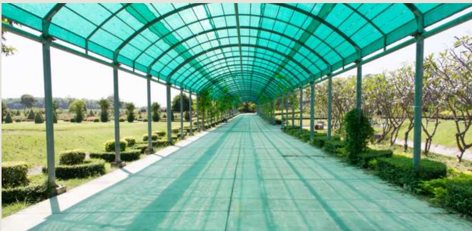
Figure 33. Steel walkway covered with shading net. Source: Getty Images.
