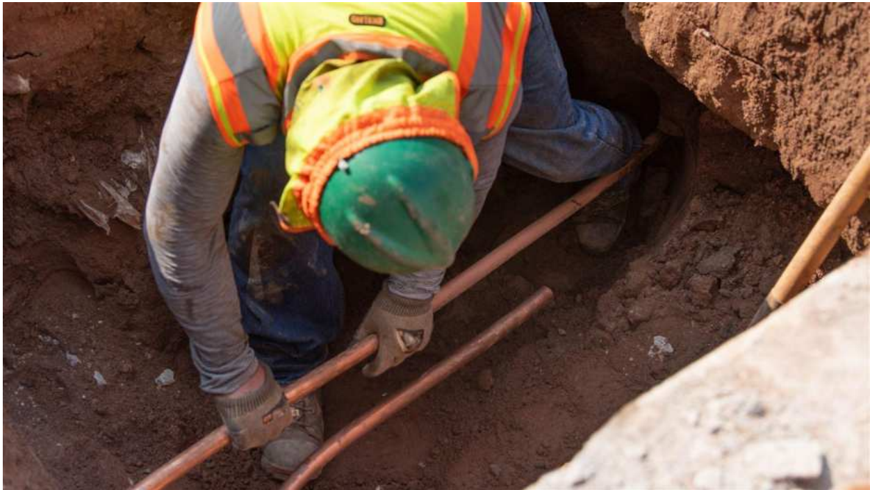
Figure 9. Worker installing copper pipes underground ( CDM Smith, 2024 )
