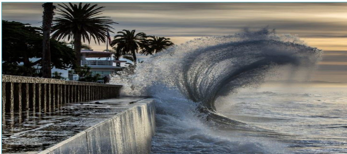
Figure 4. Seawall in Santa Barbara, California
