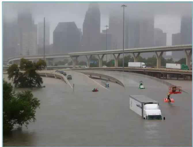
Figure 2. Flooding during Hurricane Harvey
