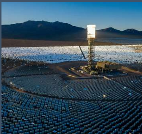
Solar Electric Generating System via Noah Berger
