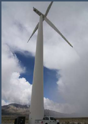
Spring Valley Windfarm via Gretchen Baker
