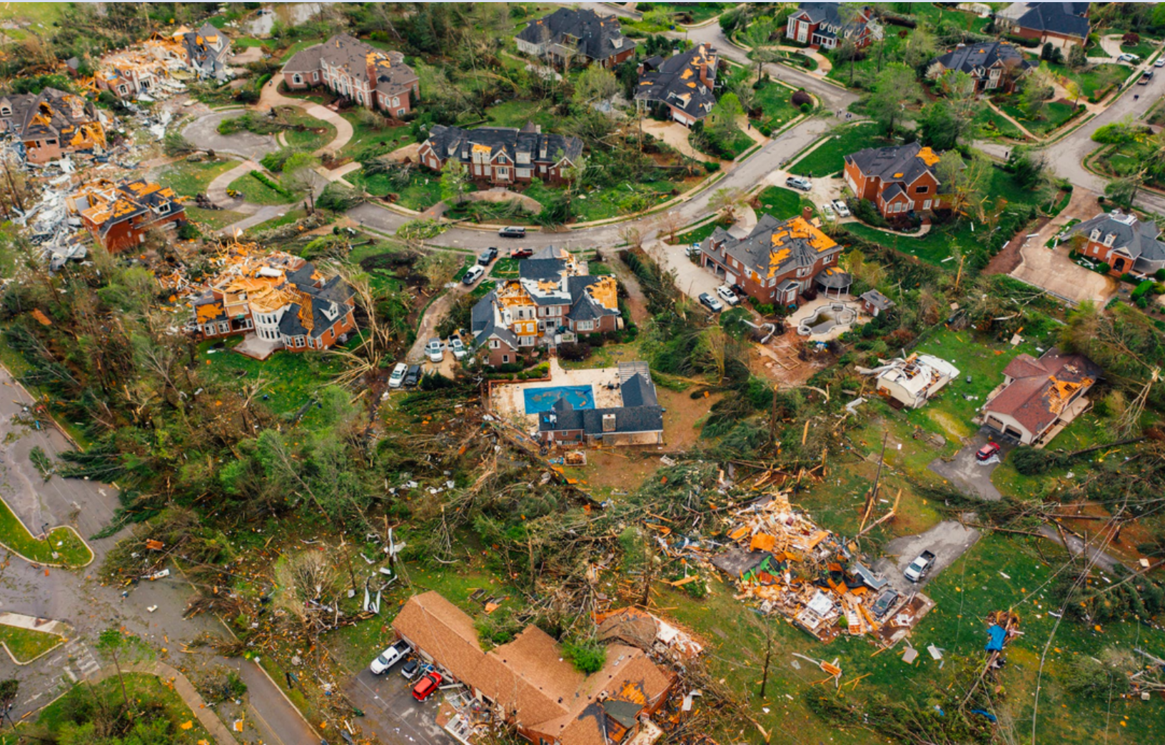
Photo highlighting extreme storm damage Source: Kelly, Pexels
