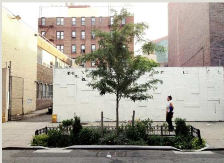
Bioswale in NYC
