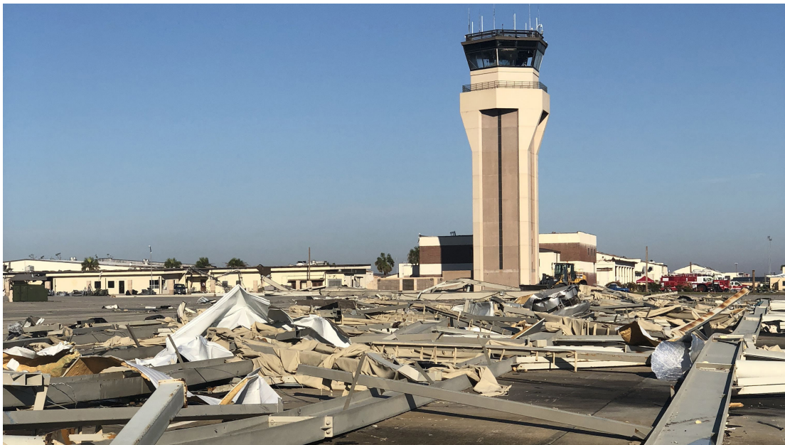
Figure 2: Tyndall Air Force Base after Hurricane Michael 2018
