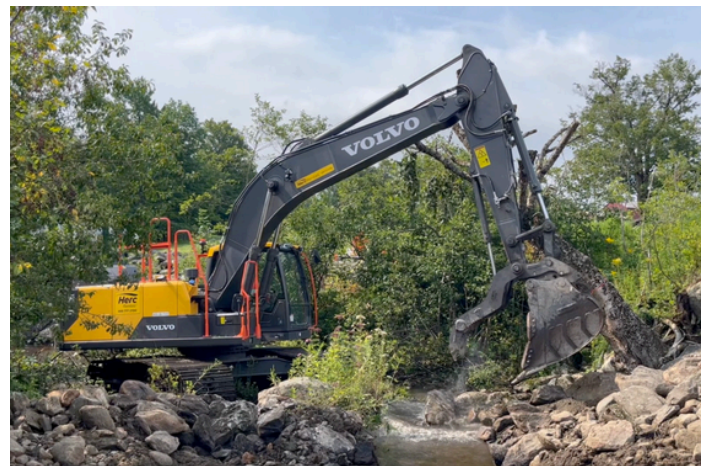
Removal of an old mill dam, Beaver Brook Dam, in Wilmington Vermont by the Connecticut River Conservancy
