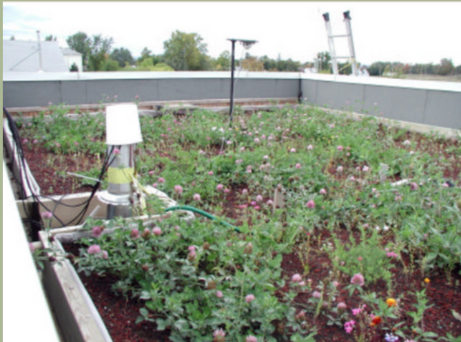
Figure 1: Ottawa Rooftop Garden on NRC building. (Source: Government of Canada) [113]
