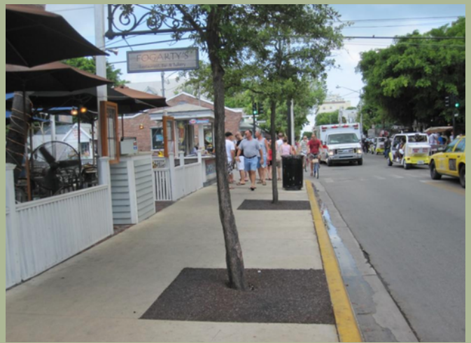
Figure 4.1: Tree pits substitute impermeable surfaces for permeable ones [104].
