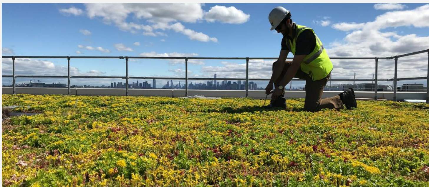
Maintaining a green roof in New Jersey. Image: Sempergreen
