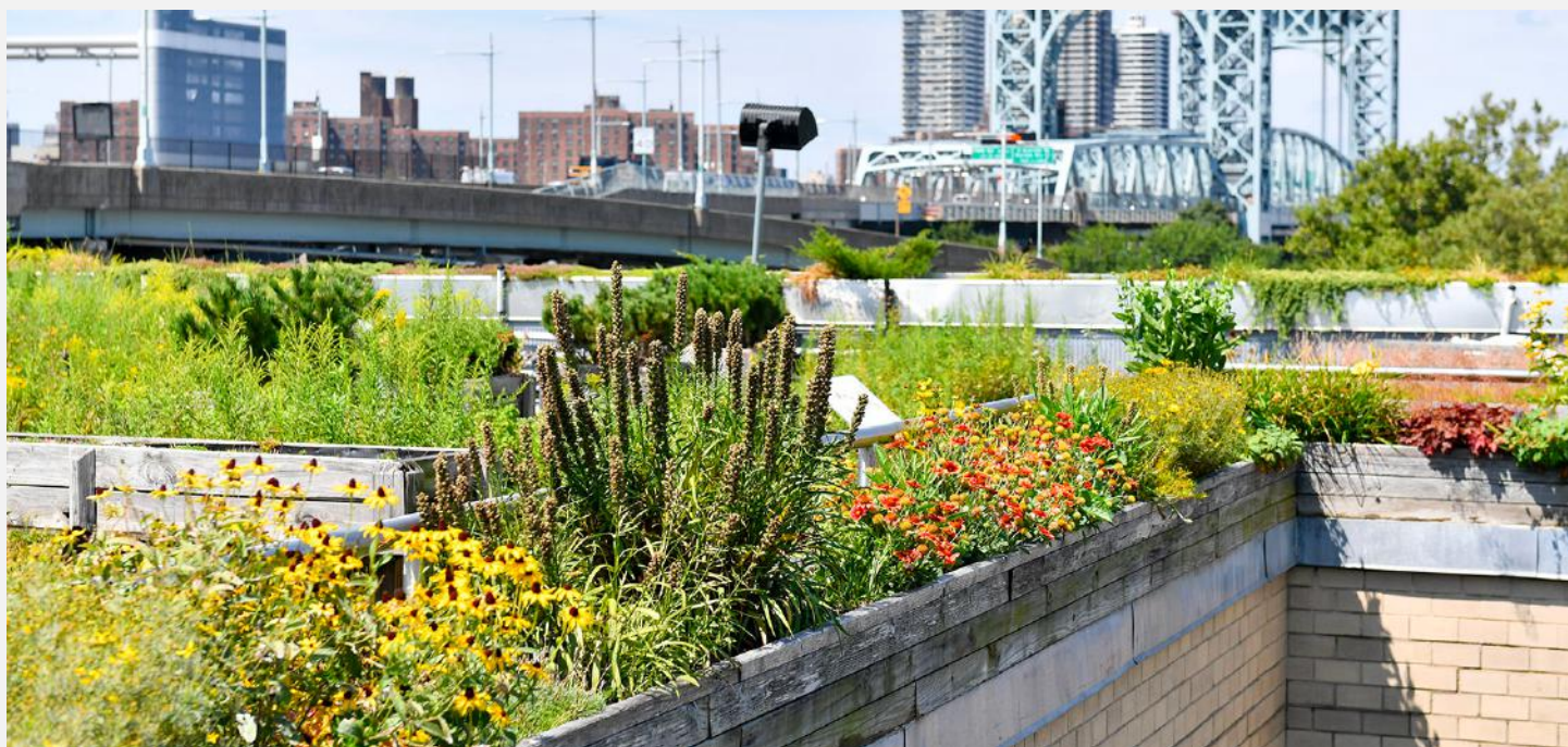
Green roof on NYC Parks' Five Borough Administrative Building. Image: NYC Parks
