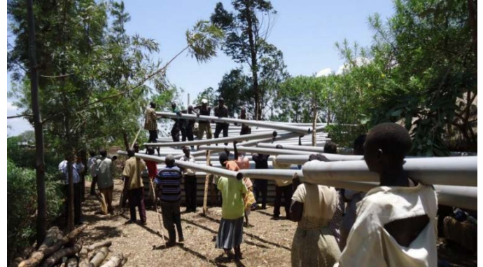
Villagers assisting the construction of the gravity flow scheme in Sanzara, Uganda Photo credit: IUCN
