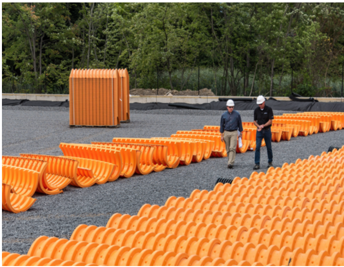
Figure 1.9: The plastic chamber storage detention basin system used in the Eastridge High School, NY (LaBella)
