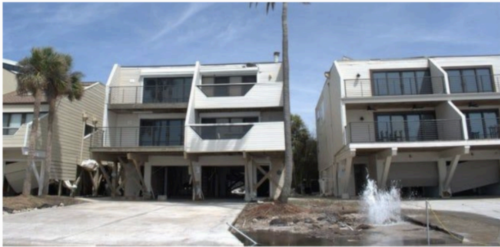
Figure 11: Damage to balconies, facades and other non-structural elements of elevated buildings in Steinhatchee, FL (Source: Kathleen Flynn, Reuters)
