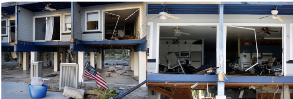
Figure 11: Damage to balconies, facades and other non-structural elements of elevated buildings in Steinhatchee, FL (Source: Kathleen Flynn, Reuters)
