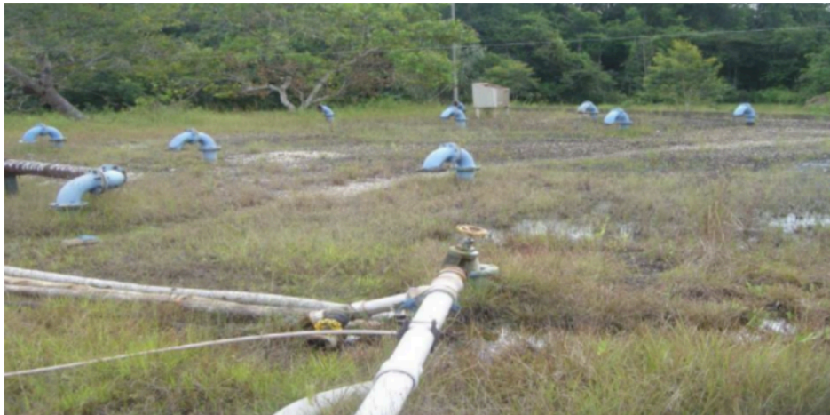
Appendix L – Photo of R05 illustrating the surface being overtaken by vegetation(PMSB)
